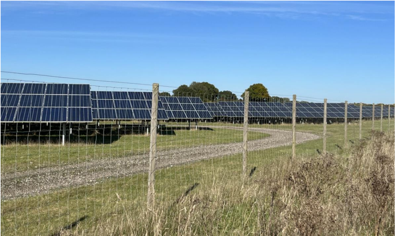
Plate 2-8: Typical crushed stone access track laid on hardcore and geotextile
