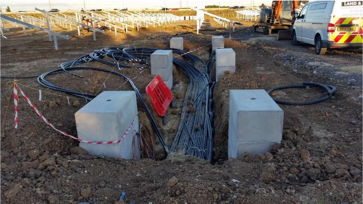
Plate 2-6: Example underground cable installation
